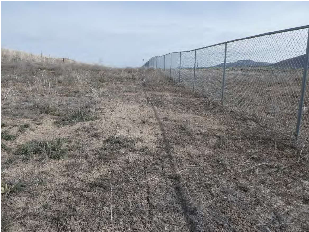
Fencing along the East Waste Repository boundary
